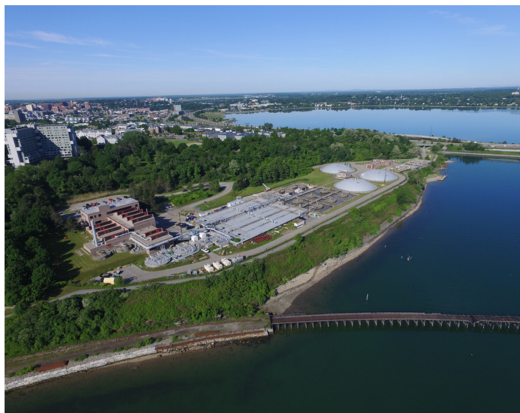
Aerial image of the East End Wastewater Treatment Facility.
