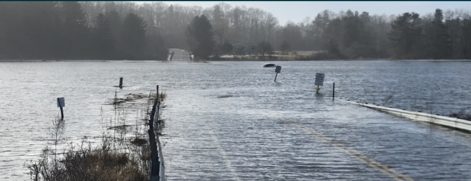
Storm surge across Sawyer Road. Photo by PPH.
