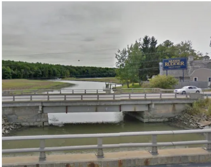
Image of US 1 bridge across Cousins River. Photo by PPH.
